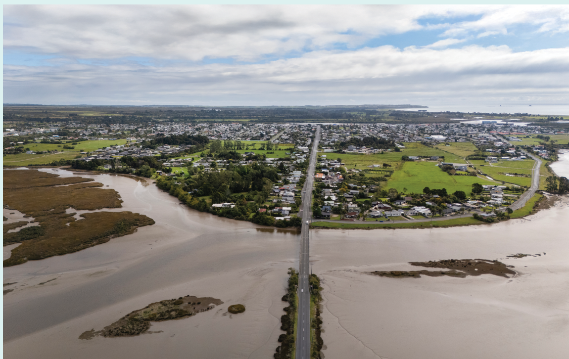
The bridge crossing the Orowaiti River at Westport.
